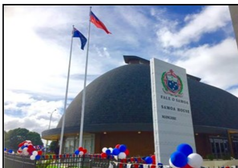
The new Samoa Consulate Fale Building at Mangere
